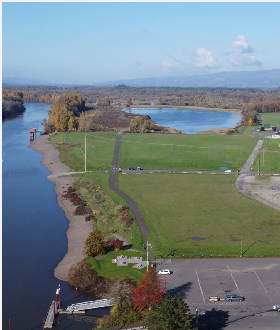
Bird's-eye view of the project site.
