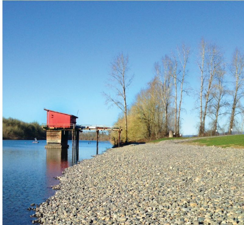
The pumphouse, located near the north end of the project site.
