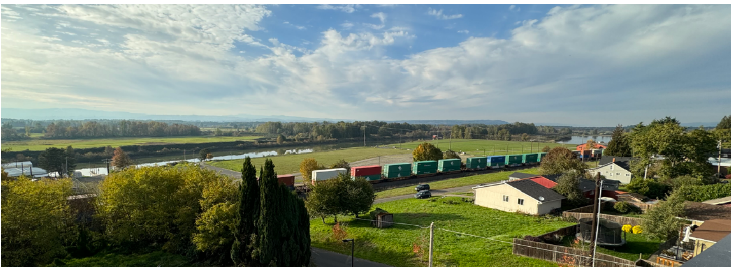
View of the project site from the Port office.
