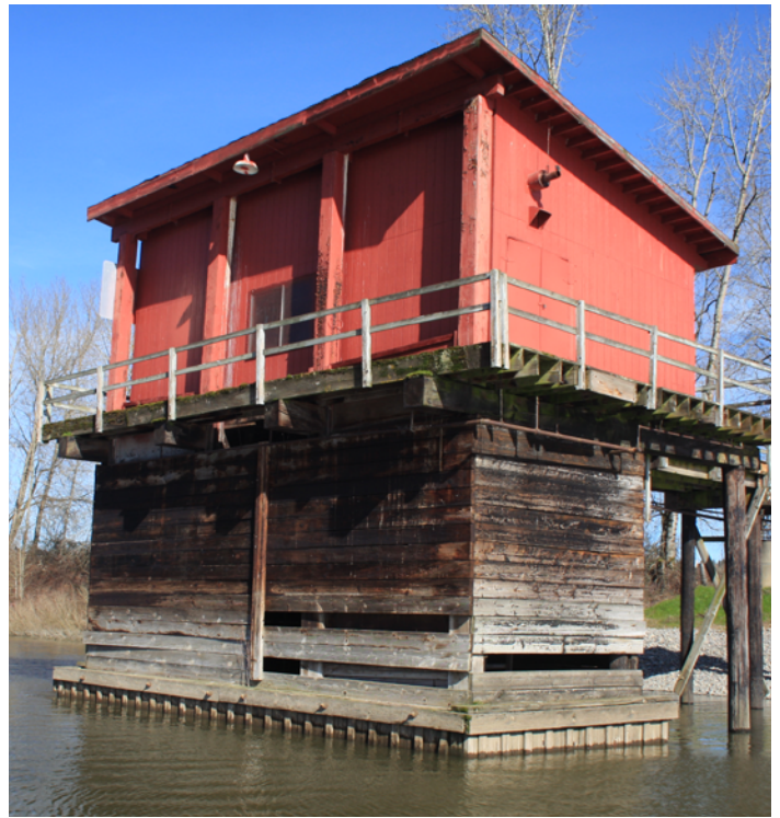
The pumphouse (front view) taken from the water.
