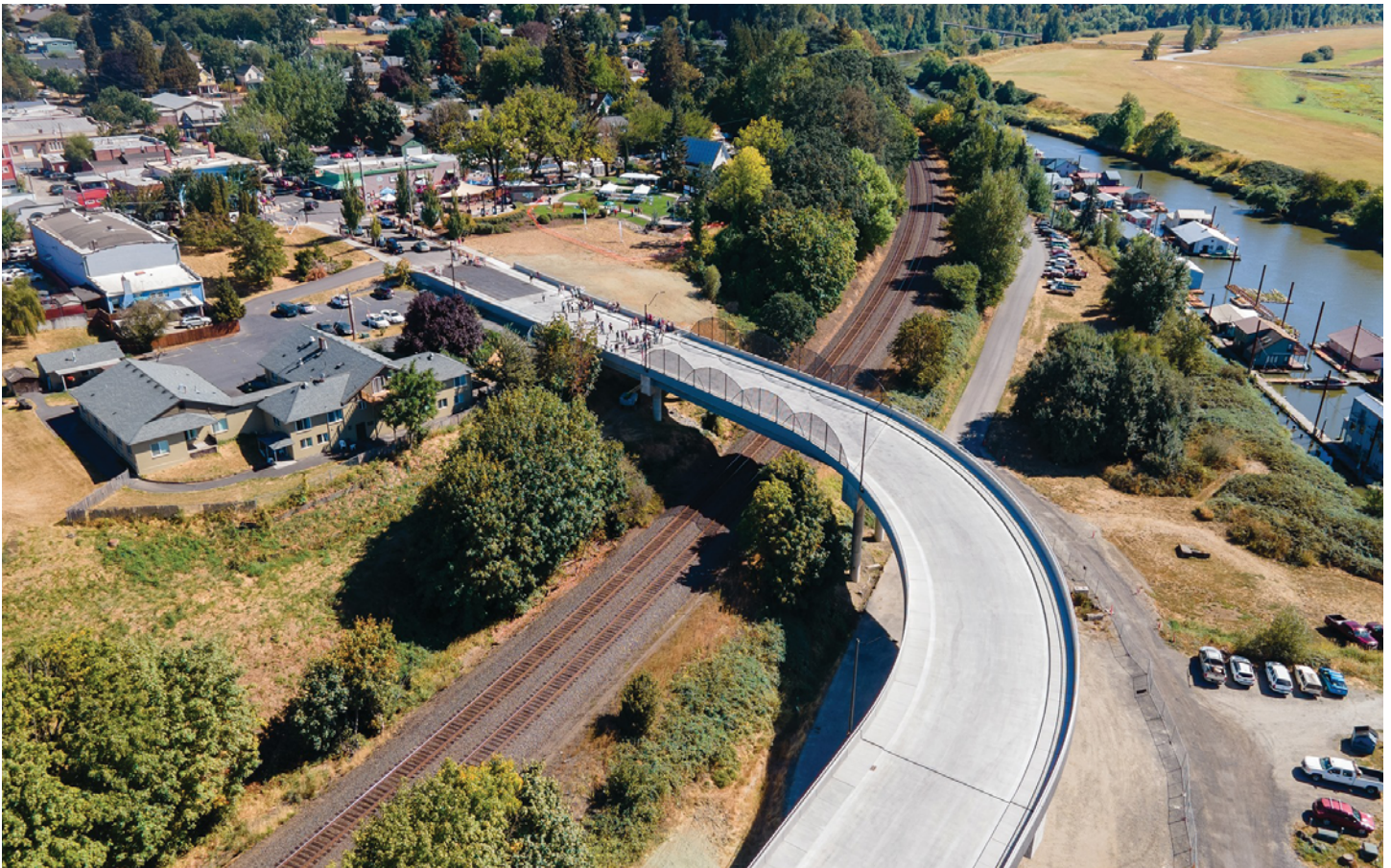
Pioneer Street overpass.
