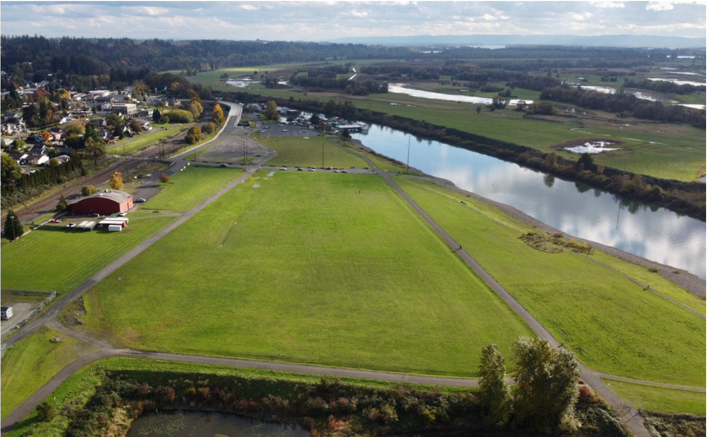
Bird's-eye view of the project site.
